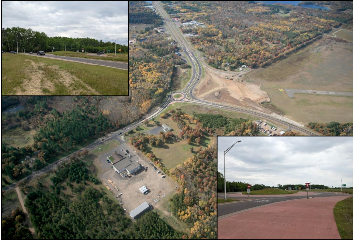
Photos: Top Inset, WIS 35 / 70 Intersection Roundabout (facing south); Center, Aerial Image of WIS 35 / 70 Intersection Roundabout; Bottom Inset, WIS 35 / 70 Intersection Roundabout (facing west) (Photo Source: Top Inset, NWRPC; Center, WisDOT; Bottom Right, NWRPC)
