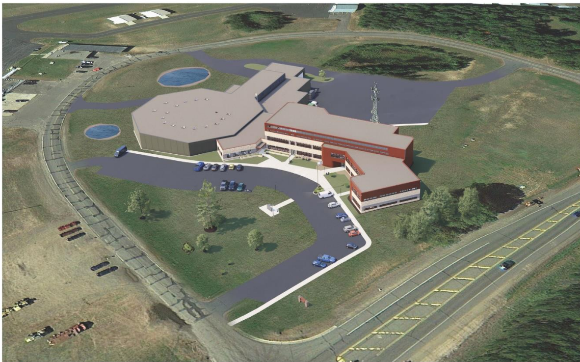
Aerial View Looking Northwest Burnett County Public Safety Facility
